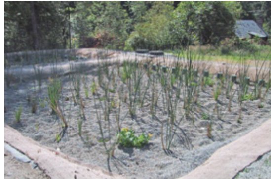
Living Machine's third-generation systems will use wetland cells as the primary means of filtration.
